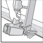
Engage the nailer onto the tongue-side of the board. Drive the nail no further than 1 in (2.5 cm) from each end of the board and 4 to 6 in (10 to 15 cm) from either sides of the center.
